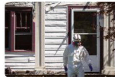
A qualified person must perform a risk assessment and wear appropriate PPE prior to entering a structure.
